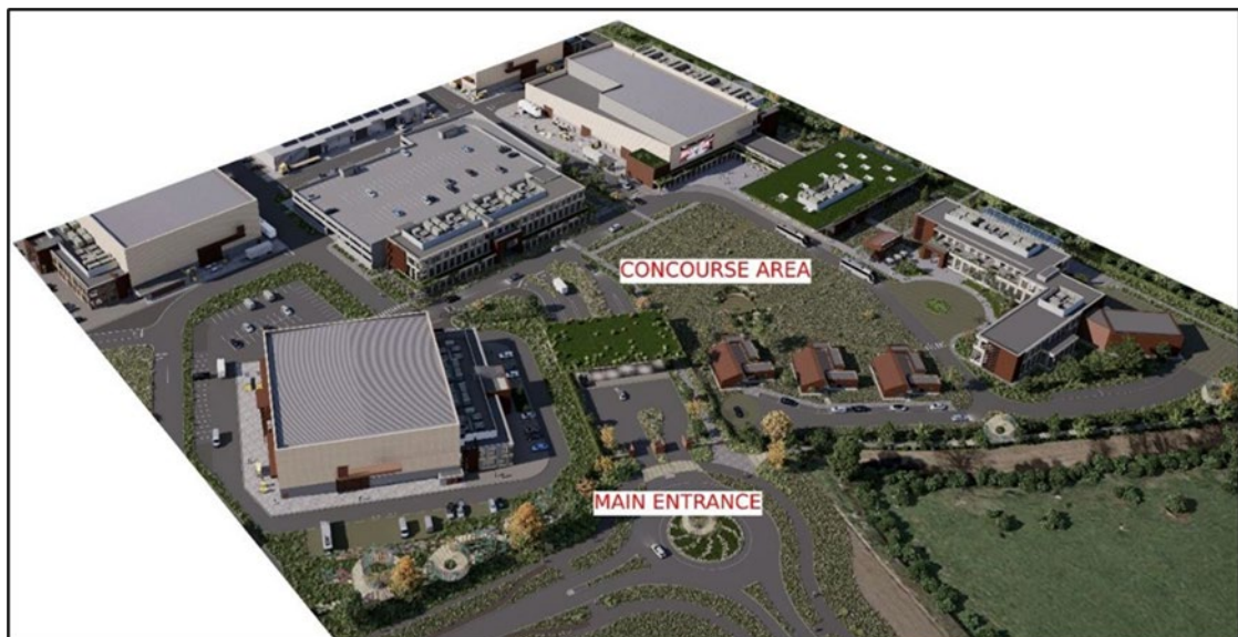
Figure 3.22: View from South-East of buildings defining the main concourse area.
