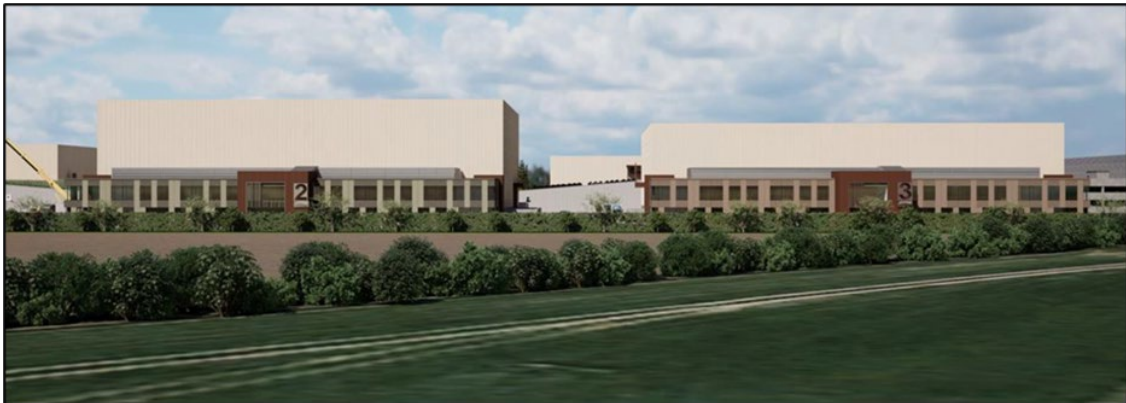
Figure 3.28: View of "Back of House" Stage Office elevations along the southern boundary.
