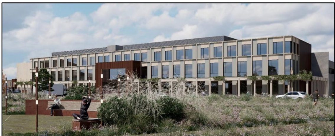
Figure 3.9: View of Production Office from the northeast.
