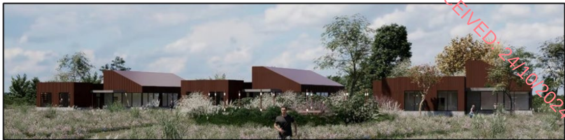
Figure 3.38: View of Production Suites from East.
